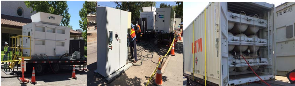
Figure 3: CNG Capture portable generator, mobile compressor, and CNG trailer 60
