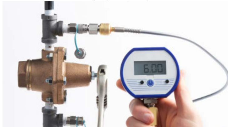
Figure 5: Differential pressure test using pete's plug 62
